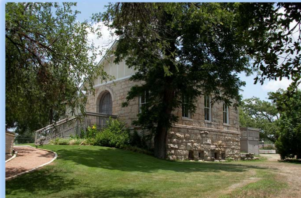
Brackenridge Pump House #2, 1885 The Borglum House
