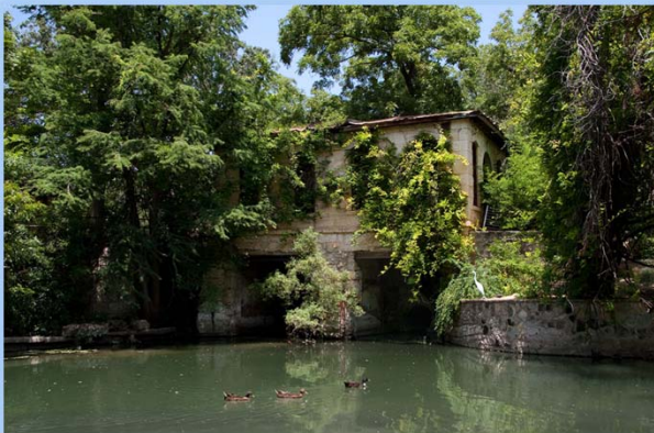
Brackenridge Pump House #1, 1877
