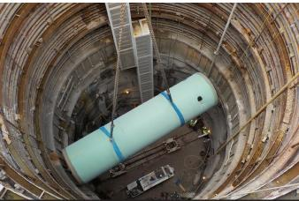
Construction crew lowers pipe into place for installation in a tunnel beneath the San Marcos River.
