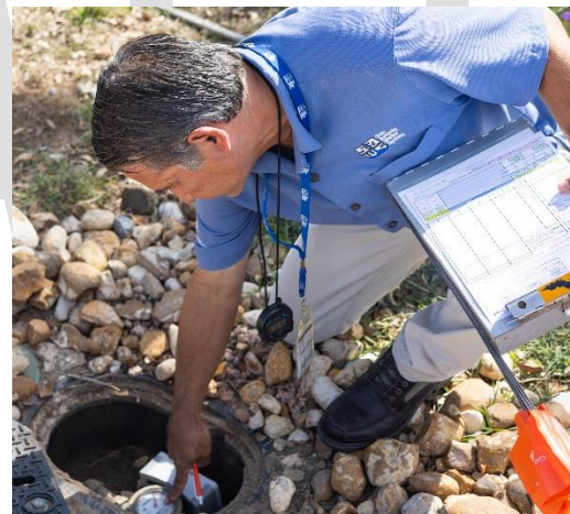
A SAWS Consultant reading a customer meter to check for irrigation flow.
