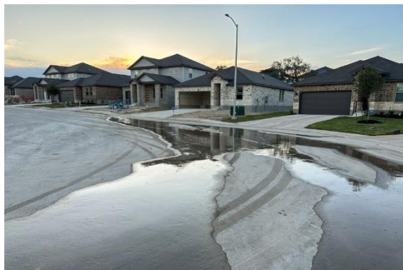
Image: Water run-off from improperly working irrigation system pools in the street. This amounts to water waste under SAWS' Conservation rules.
