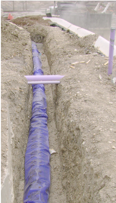
Figure 10.3 Purple sleeve around buried pipe and pipe with integral purple color
