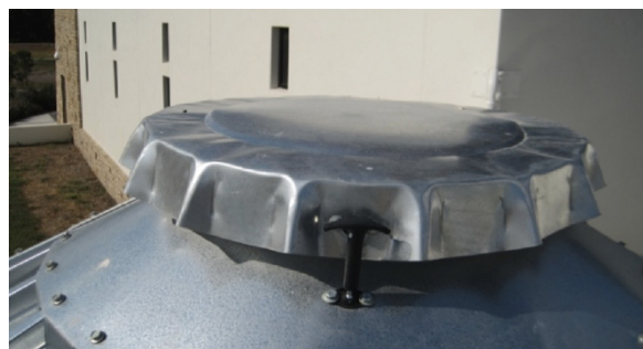
Figure 9.10 Round tank access port with locking lid
