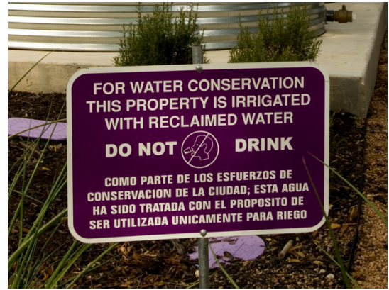
Figure 10.9 Sign identifying reclaimed and recycled water combined in a storage tank
