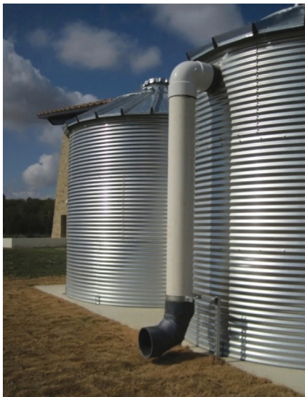
Figure 9.12 Tank overflow pipe
