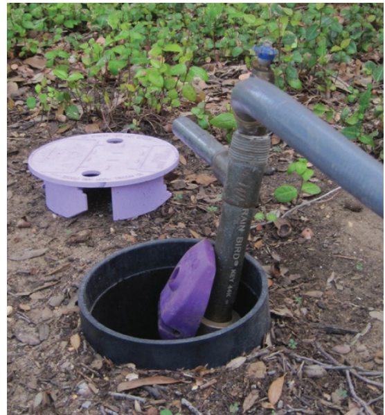
Figure 9.15 Purple quick-disconnect valve in purple valve box with valve key in place and connected to a compatible hose
