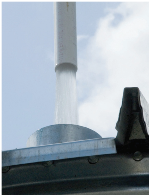
Figure 9.13 Air gap between potable or recycled make-up water and reclaim storage tank
